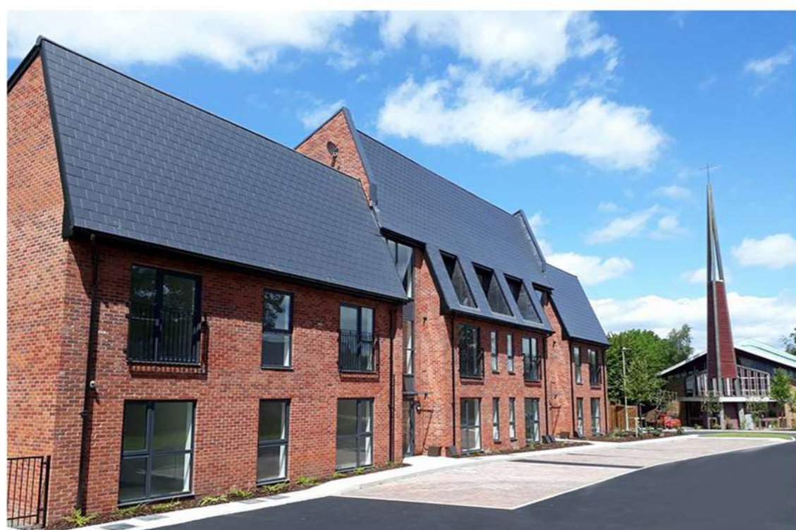
ST ALDATES - BM3 & ROOFTOP
