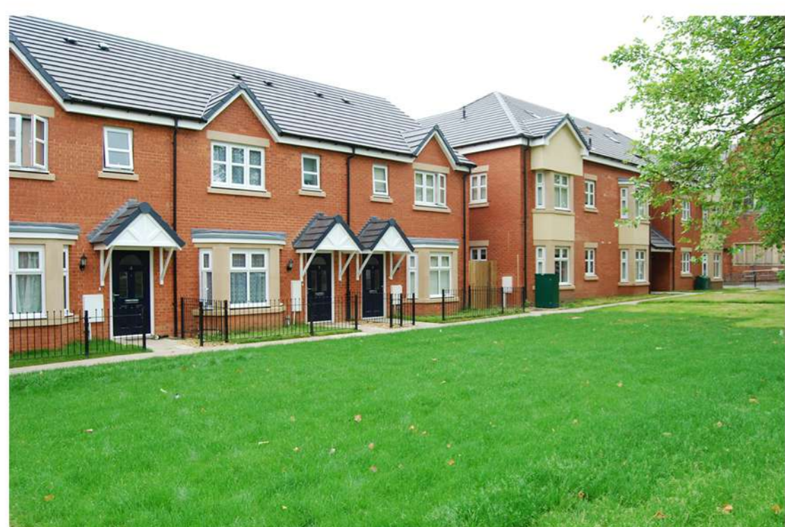
FRAMPTON CORNER - BM3 & ROOFTOP
